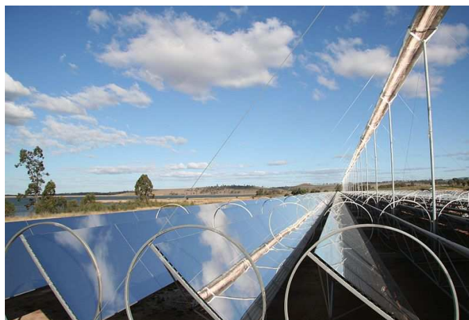
Linear Fresnel mirrors direct the rays towards the focal point, top right.
