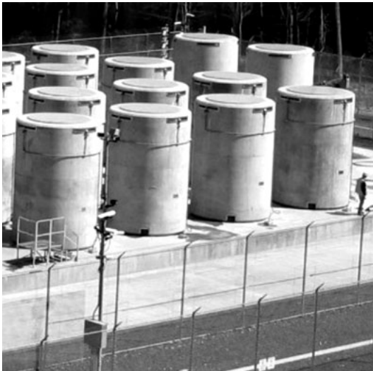
Figure 1.6: Dry cask storage at the Connecticut Yankee spent fuel storage facility. There are 43 dry storage casks on the site, of which 40 hold spent fuel and three store high-level radioactive waste. Source: Connecticut Yankee Atomic Power Company.
