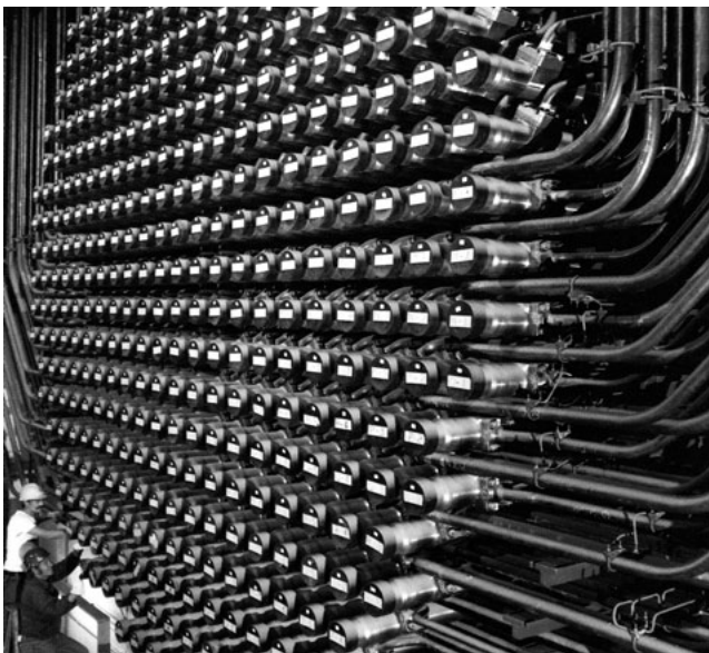
Figure 14.2: CANDU reactor face showing end fittings of the pressure tubes to which the refueling machine attaches. Source: Atomic Energy of Canada Limited.
