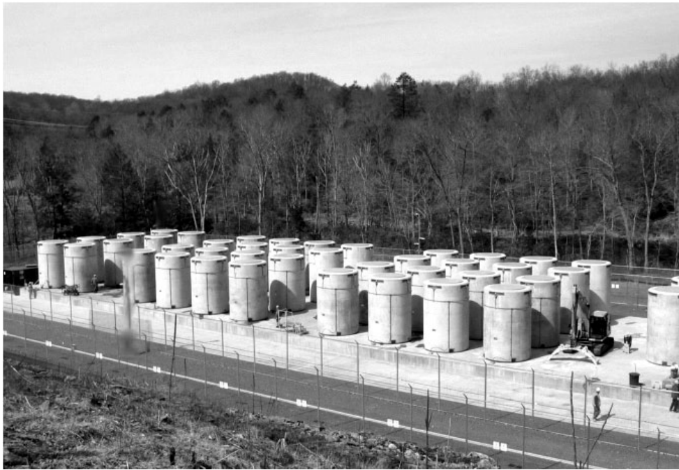
Figure 10.1: Dry cask storage in the United States. Forty one casks contain 412 tons of spent fuel, the lifetime discharges from the Connecticut Yankee
