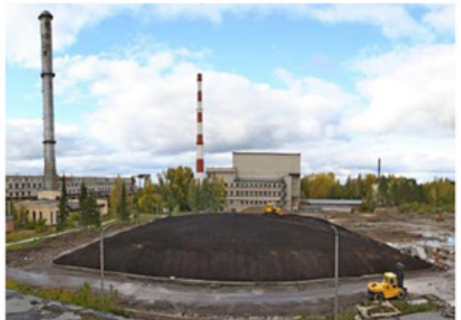
Fig. 4. View of PUGR EI-2 above ground facilities before (left) and after entombment (right)
