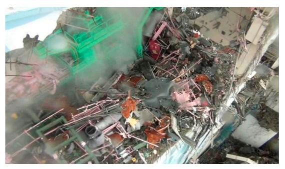
Figure 1.11 - Debris in the spent fuel pool of Fukushima-Daiichi 4 after the hydrogen explosion, with steam rising. Source: TEPCO.
