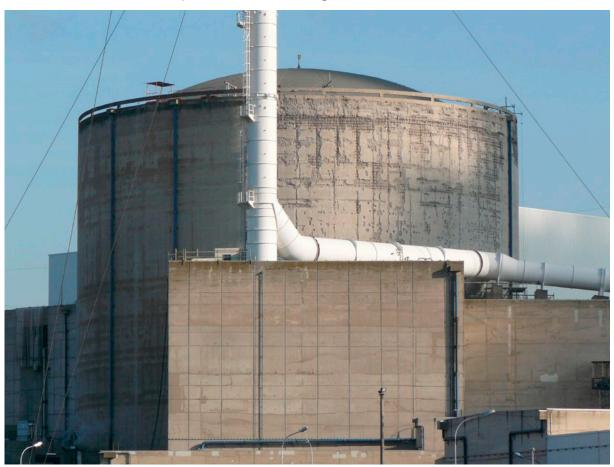
Figure 1.8: - Ageing damaged outside wall of the reactor building at the Belgian nulcear power plant Tihange. (© Alain Vincent/Greenpeace)
