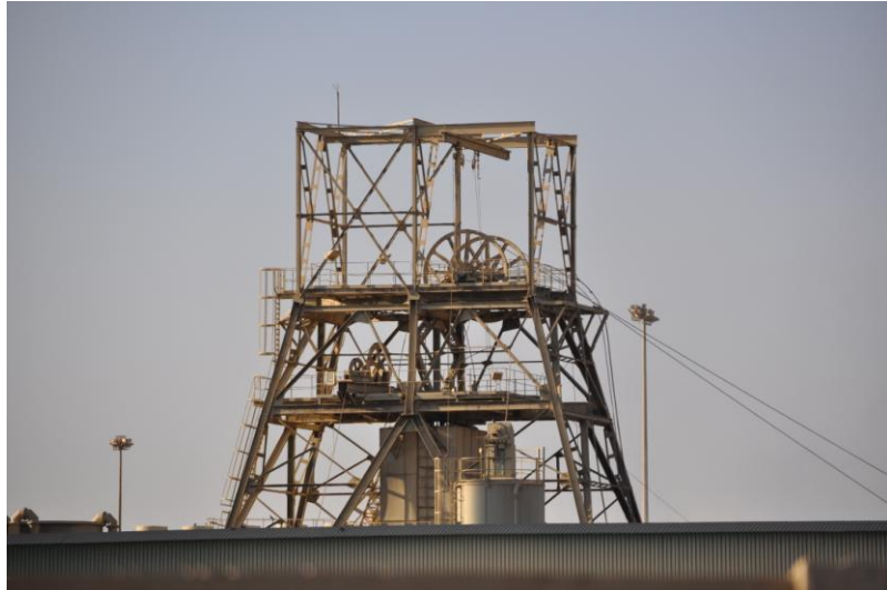
Above-ground Constructions at Ezulwini's Underground Mine
