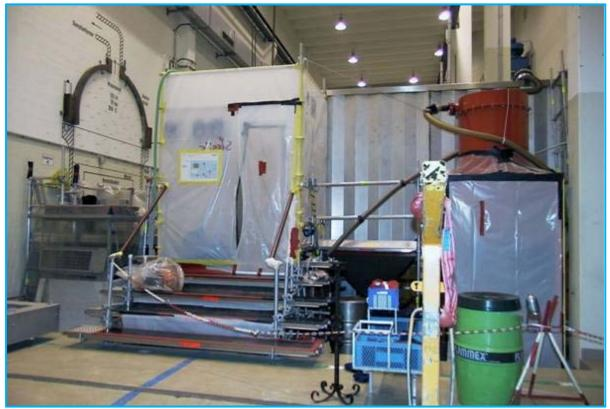
Figure 6-6: Blasting caisson at NPP Kahl
