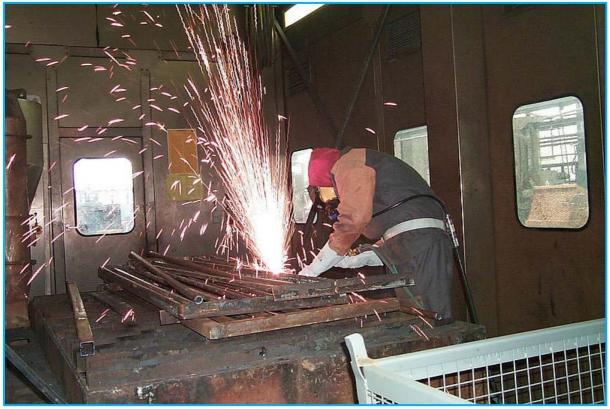
Picture by courtesy of EWN Figure 6-3: Thermal Cutting
