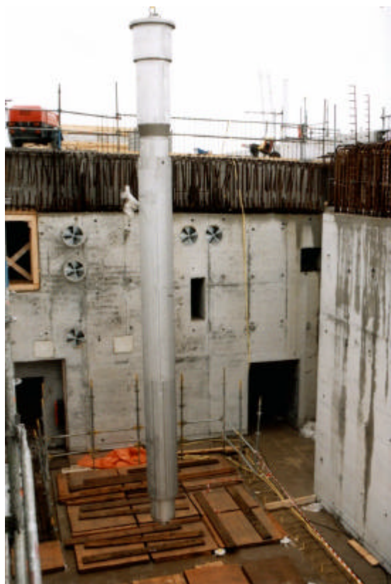
Figure 4. Emplacement of the wells during construction
